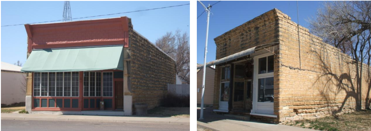
Figure 16: These one-story commercial buildings in Sylvan Grove, Kansas are constructed of limestone post-rock. Both feature Mesker Brothers Iron Works elements—the building on the left sports a pressed metal cornice (with fleur-de-lis) and the building on the right features cast-iron columns on either side of the traditional storefront. Photos taken by the author, March 16, 2009.
