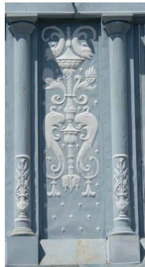
Figure 14: The stylized dolphin panels on this Mesker Brothers façade were installed upside down. The image on the left exhibits the incorrect installment of the panels, with the pair of dolphins upside-down. The image on the right shows the correct way the panels should appear, with a dolphin on each side and a torch just above the head of each figure. Photo on left was taken by the author, the image on the right is from the Identification Guide, Illinois Historic Preservation Agency, www.gotmesker.com (Accessed March 31, 2009).
