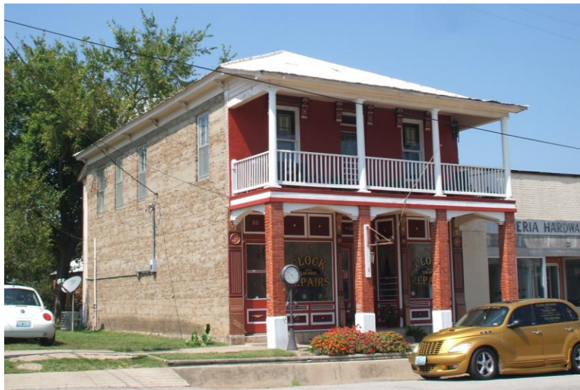
Figure 15: Located in Iberia, Missouri, this commercial building is constructed using poured concrete and is adorned with George L. Mesker & Co. Cast Iron elements. Photo taken by author.
