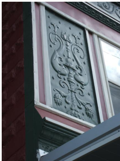
Figure 14: The stylized dolphin panels on this Mesker Brothers façade were installed upside down. The image on the left exhibits the incorrect installment of the panels, with the pair of dolphins upside-down. The image on the right shows the correct way the panels should appear, with a dolphin on each side and a torch just above the head of each figure. Photo on left was taken by the author, the image on the right is from the Identification Guide, Illinois Historic Preservation Agency, www.gotmesker.com (Accessed March 31, 2009).
